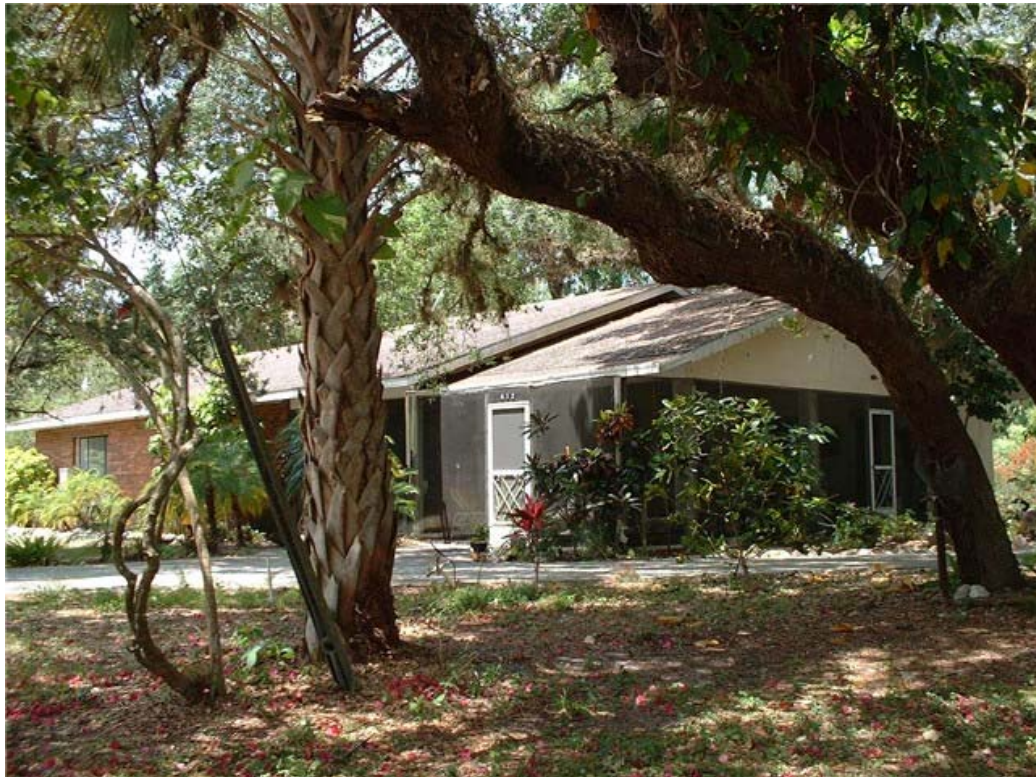
Figure 1-6. East front of Park House from Fraser Avenue.
