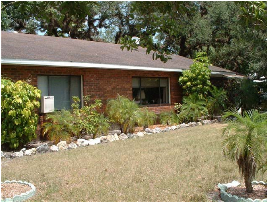
Figure 1-5. South face of Park House.
